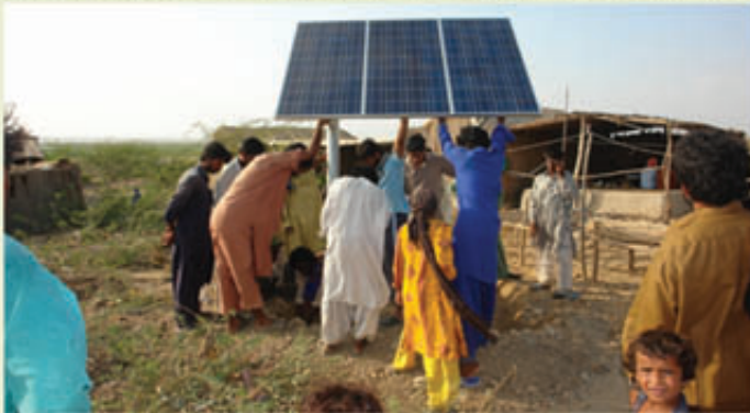
A solar panel installed at Keenjhar Lake
