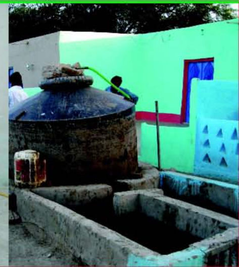
Biogas Plant
