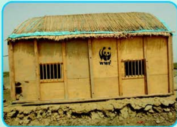
An improved hut in Hajamro Creek
