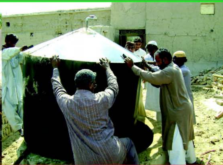
Installing a biogas plant
