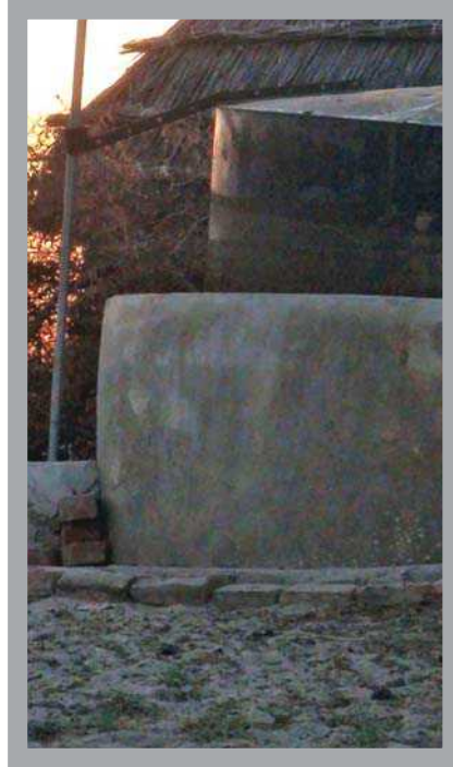
The bio-gas plant at Faqir Wanhyal Mangrio
