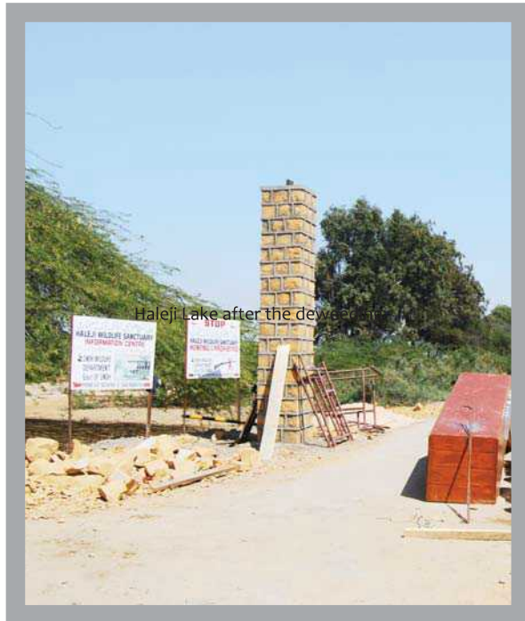
Construction of entrance gate
