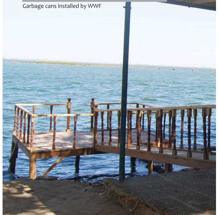
Jetty constructed for landing of boats
